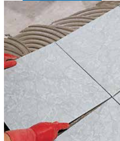
Laying porcelain tiles
