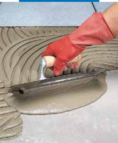
Spreading with semicircular notched trowel
