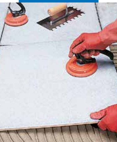
Laying large size tiles
